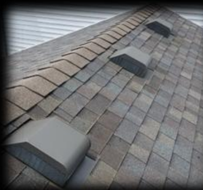
Turtle/Box Vent: Releases warm air from attic.
