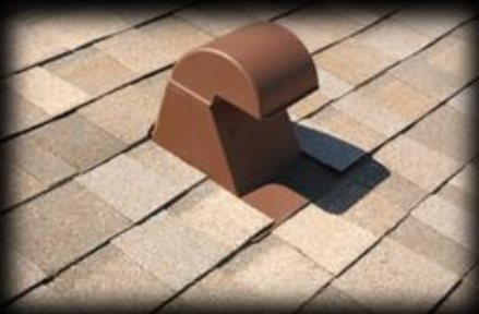
Gooseneck: Attic ventilation (kitchen hoods or dryer vents).
