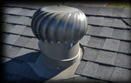
Turbine Vents: Used to draw out hot air during rainy/humid weather.
